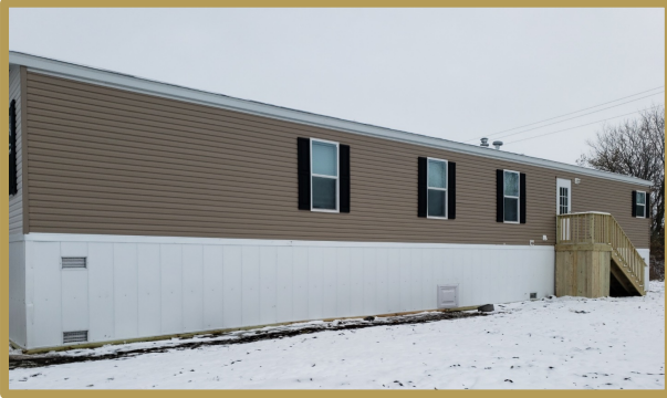
Elevated home with flood vents in skirting
